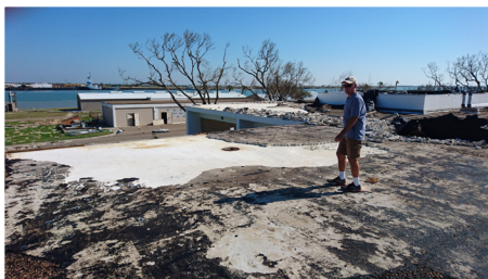
Damaged roof at the Fisheries and Mariculture Building
